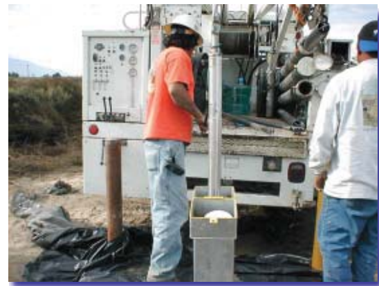
Drilling groundwater monitoring well.
