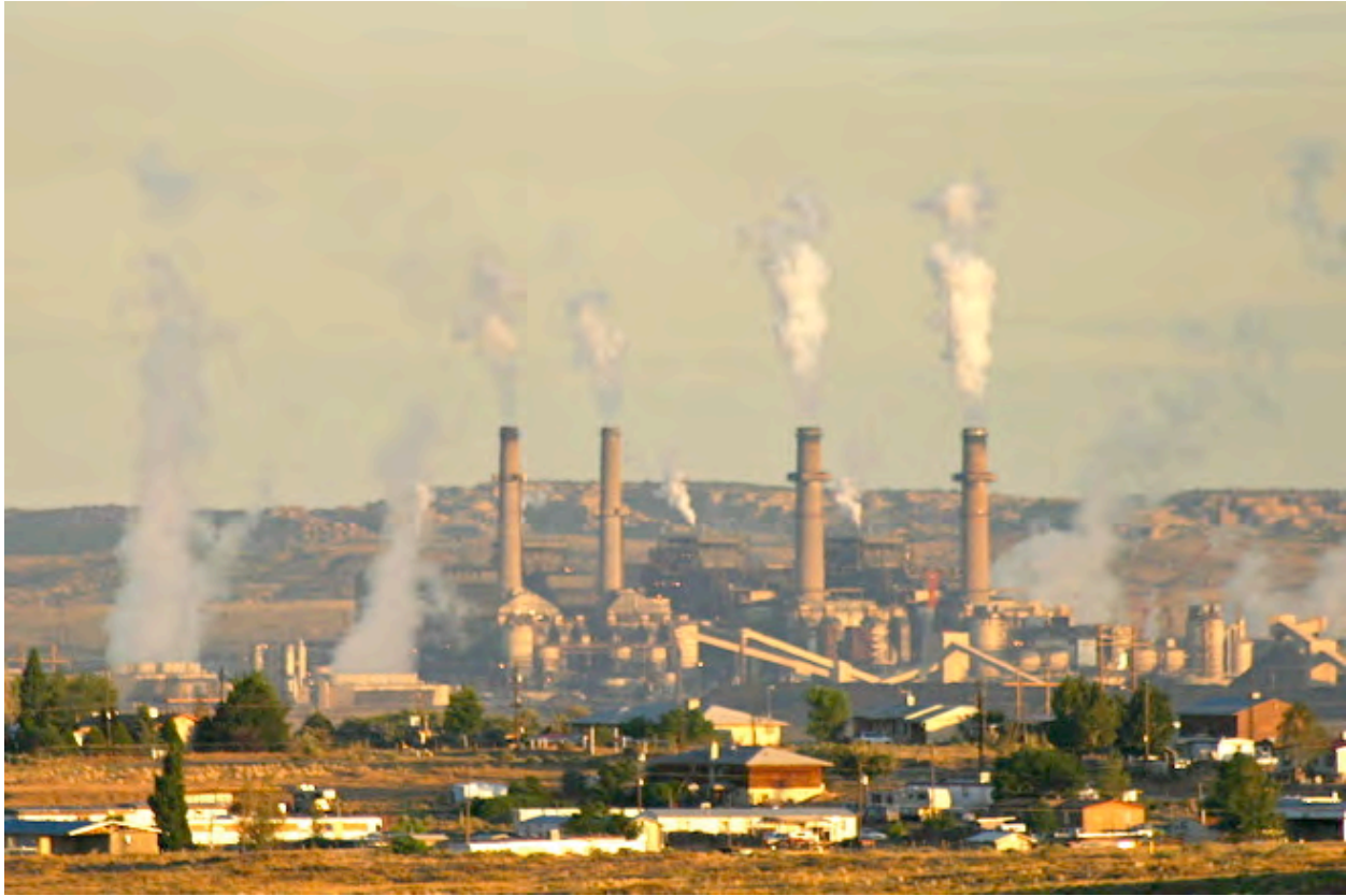
San Juan Generating Station with Homes in the Foreground (image from Flickr, jonnypeace—use of image does not imply endorsement).
