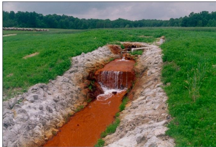
Figure 2: Anoxic Limestone Drain Outflow at the Midwestern Reclamation Site, Pike County, Indiana
