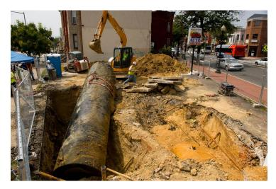
Figure 1: Underground Storage Tank Removal
