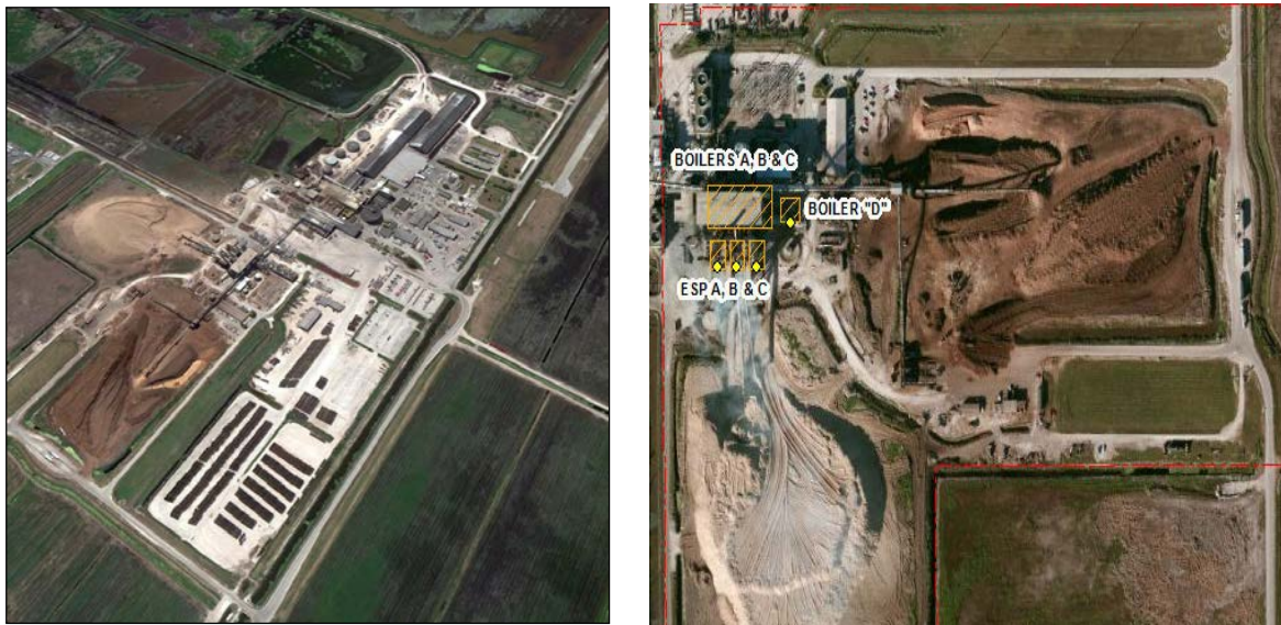
Figure 2-2 Facility Aerial View and Boiler D Location
