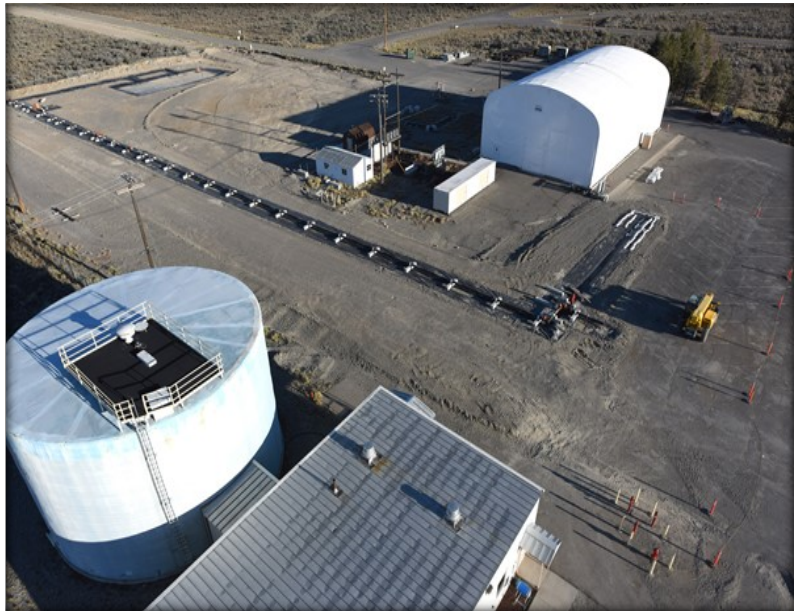
FIGURE 8. AERIAL PICTURE OF THE WATER SECURITY TEST BED.
