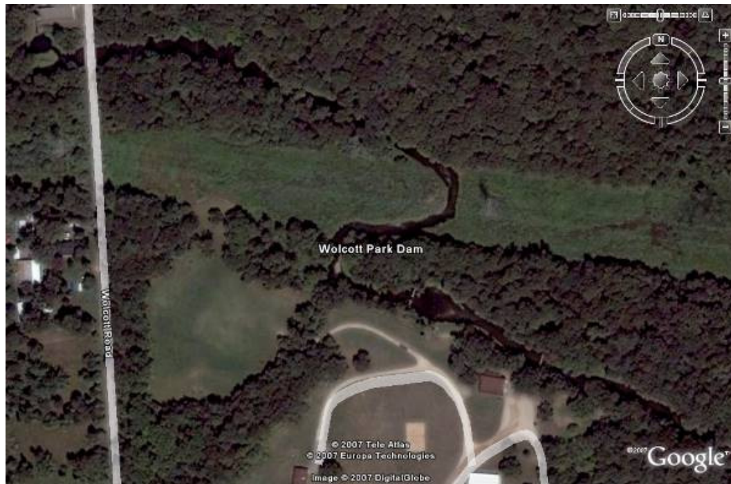
Figure 6.7. Wolcott Park Dam
