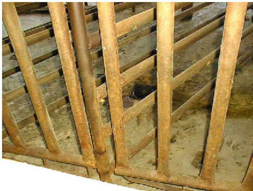
Figure 2. Floor Drain Inside of Animal Pen
