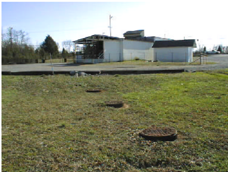
Figure 16. Location of Septic Tanks Behind Slaughterhouse and Manhole Covers
