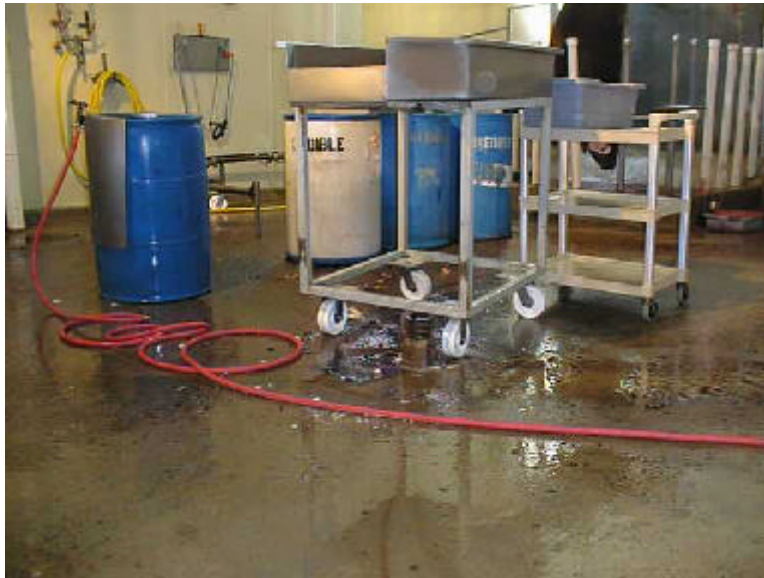
Figure 6. Floor Drain Receiving Wash Water From Equipment Washdown
