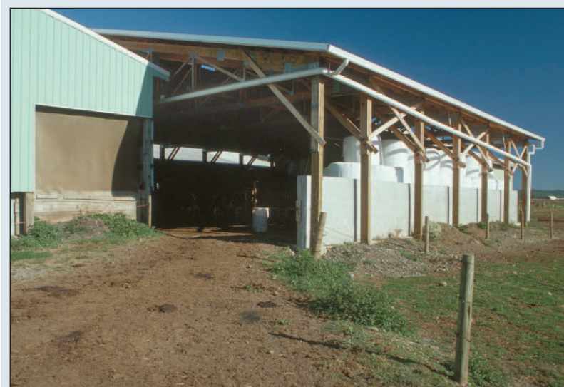
Water run-off control with the use of a gutter system at a dairy in Tillamook, Oregon. (Photo courtesy of USDA/NRCS)
