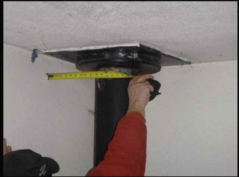
Most homes have decent ceiling penetrations
