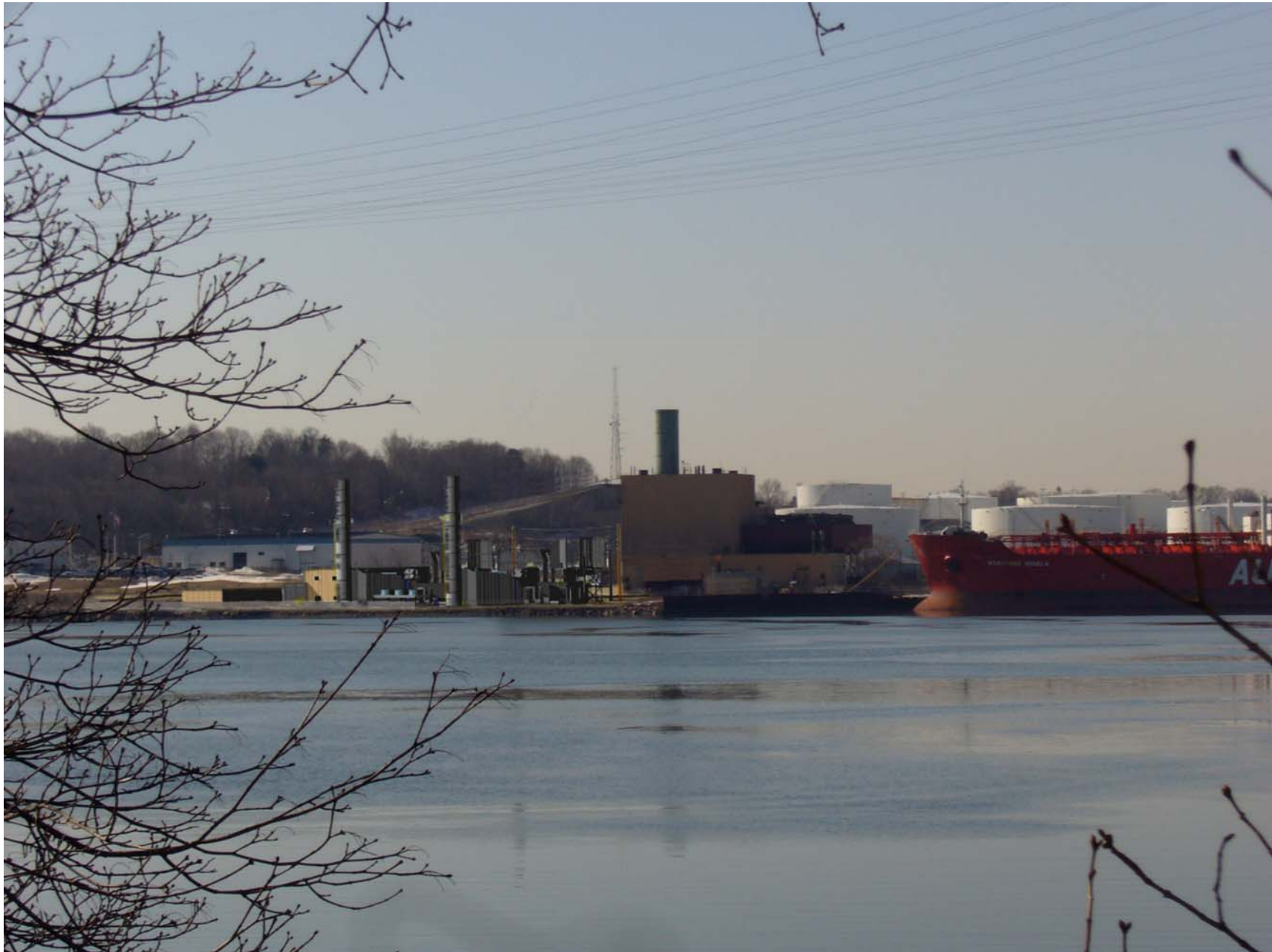
Figure 2-4 Rolls Royce Trent 60 WLE Rendering – View from Weymouth Thomas A. Watson Generating Station Braintree, Massachusetts
