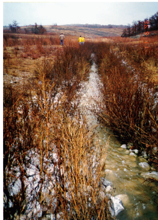
Channel for draining surface water away from containment areas at the Cherokee, Kansas site
