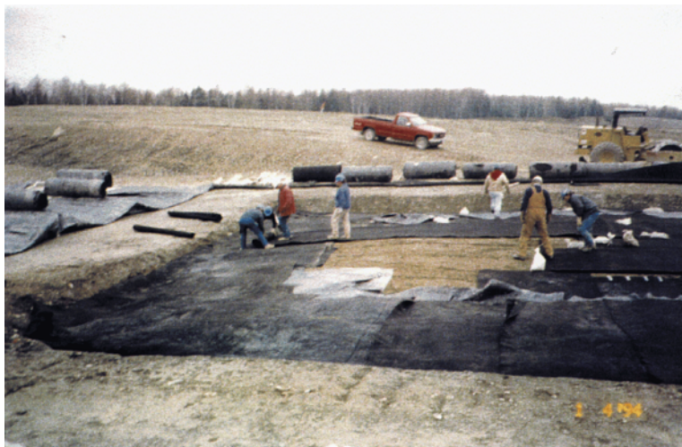
Placement of a geotextile layer at the Loring Air Force Base site
