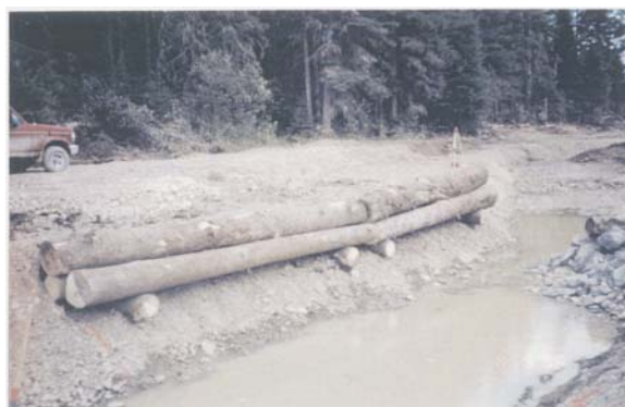
At the Loring Air Force Base site, workers used on-site materials to build a log bank
