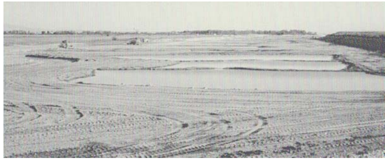
Pond area prior to remediation
