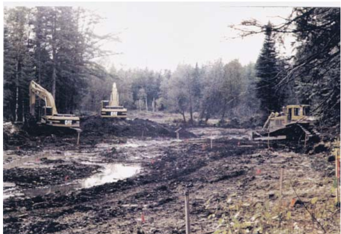
Excavating streambed at Loring Air Force Base, Limestone, Maine
