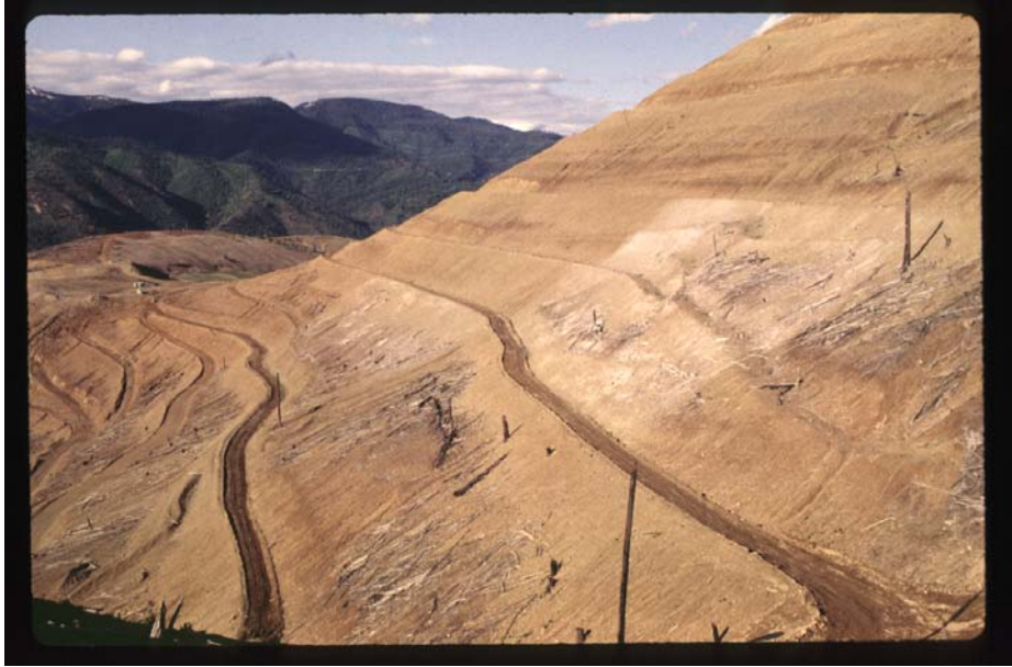
Prior to treatment denuded slopes dominated hillsides in Government Gulch. Tree seedlings, although present, are invisible in this photograph. Coarse woody debris lie on the slope to the right and toward the foreground (1997).
