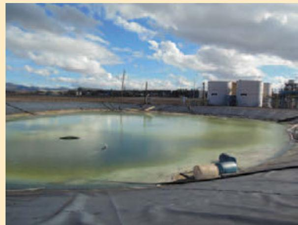
A lined pond at the Tronox facility in Henderson, Nev., still contains residual perchlorate from the pond's former use in the manufacturing process.
