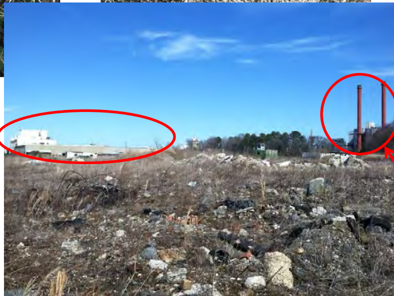
Southeastern Public Service Authority Refuse Derived Fuel facility (incinerator)
