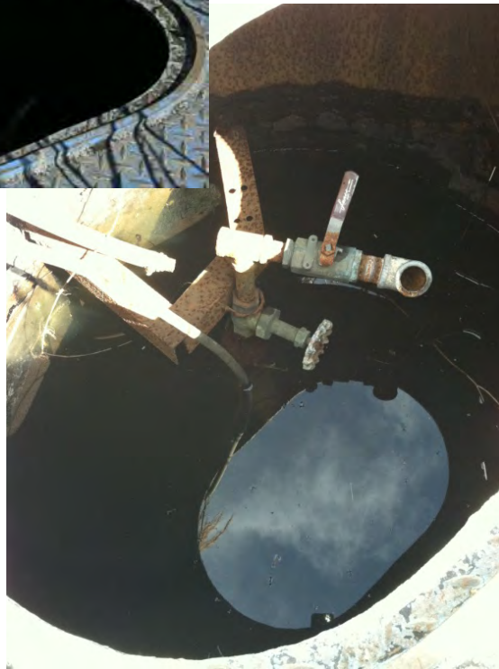
Close up inside the sump
