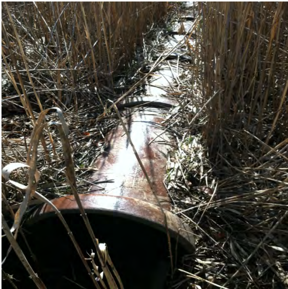
Series of pictures showing the 18"-24" pipe extending along much of the western drainage feature. The pipe is discontinuous and contains a series of junction boxes, connects and breaks along northern sections of the pipe.
