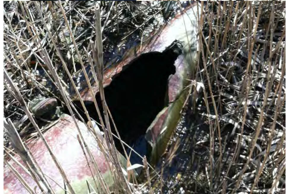
Series of pictures showing the 18"-24" pipe extending along much of the western drainage feature. The pipe is discontinuous and contains a series of junction boxes, connects and breaks along northern sections of the pipe.
