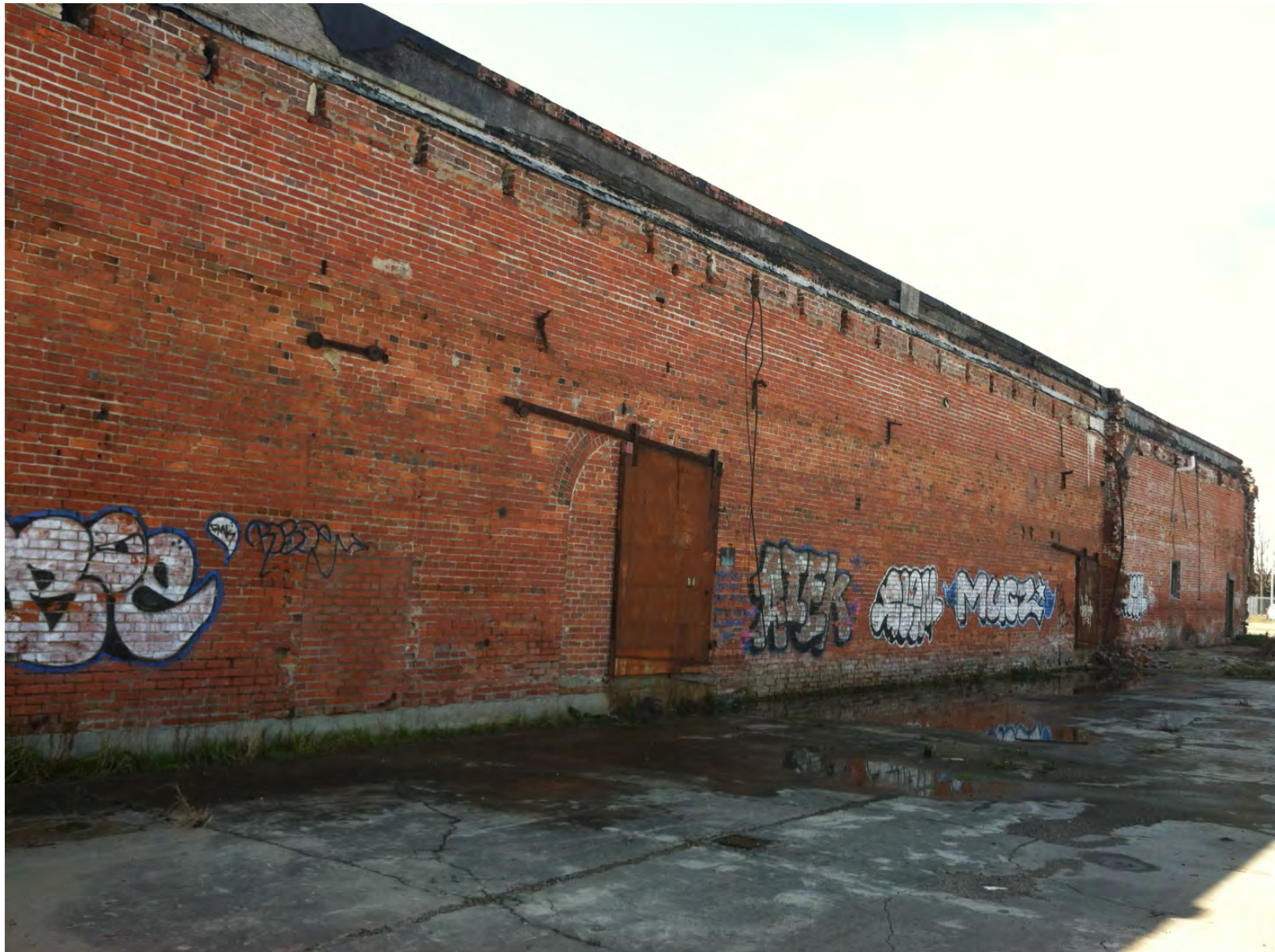
North side of main building on Peck Iron property. Looking west.
