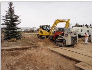
Top soil removal
