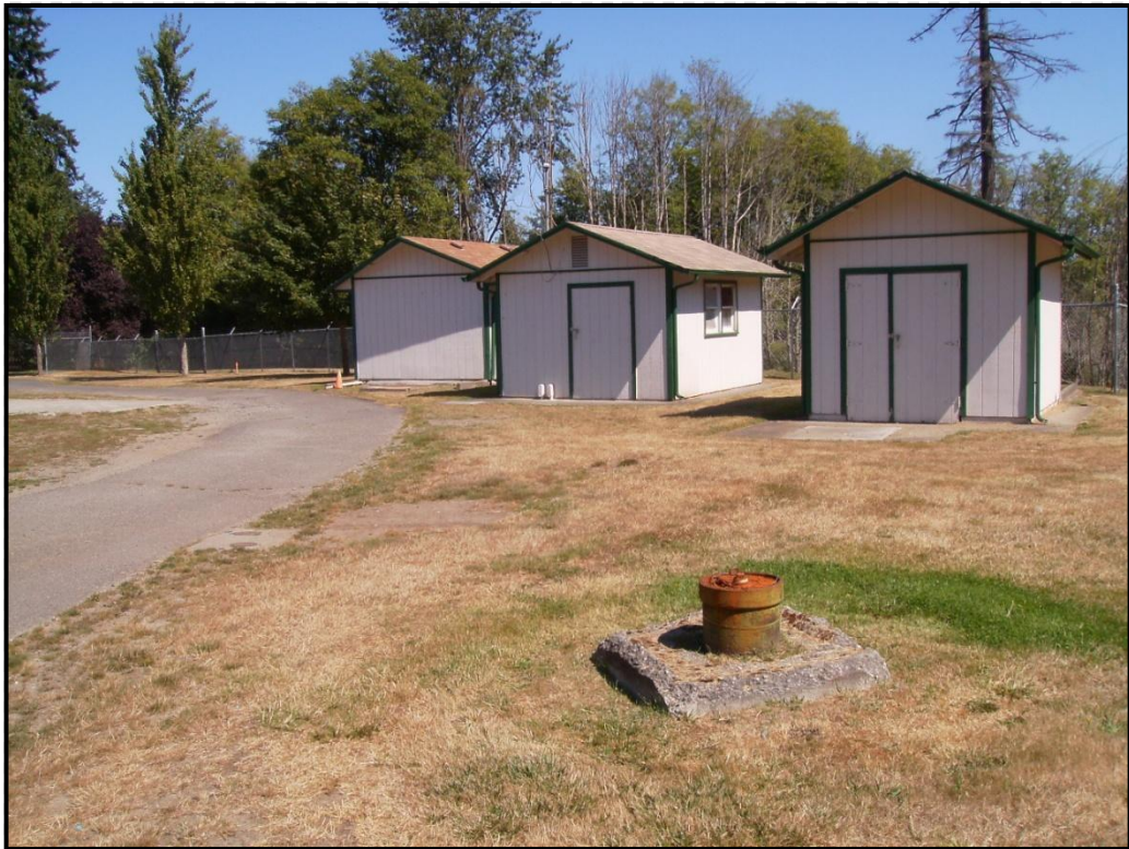
PHOTO 10: City of Tumwater Palermo Well Field – Well house structures, looking east-northeast.
