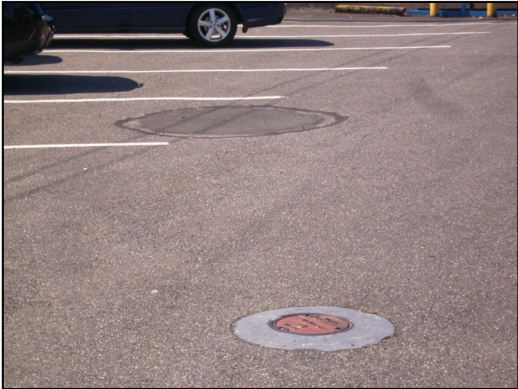
PHOTO 3: Groundwater monitoring well and abandoned large diameter feature located in the parking lot south of Southgate Dry Cleaners.
