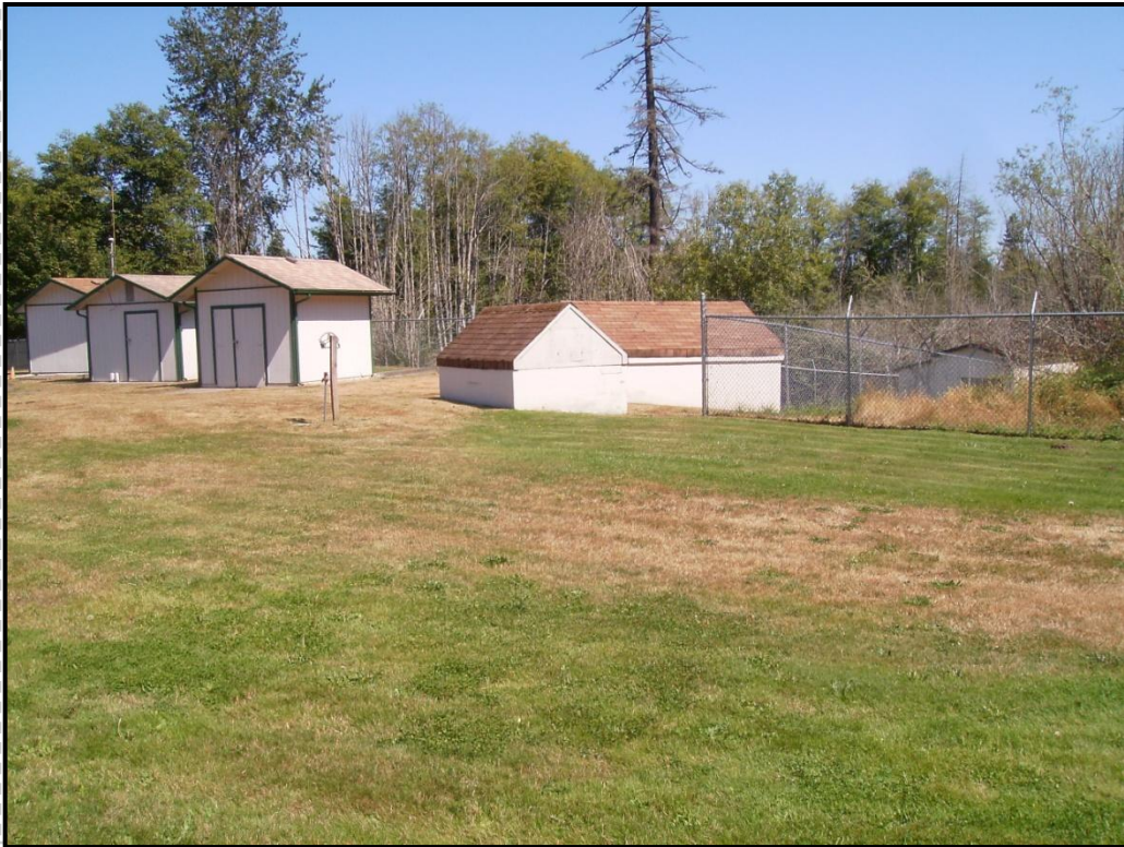
PHOTO 11: City of Tumwater Palermo Well Field – Looking northeast toward well house structures (left) and undeveloped land beyond.
