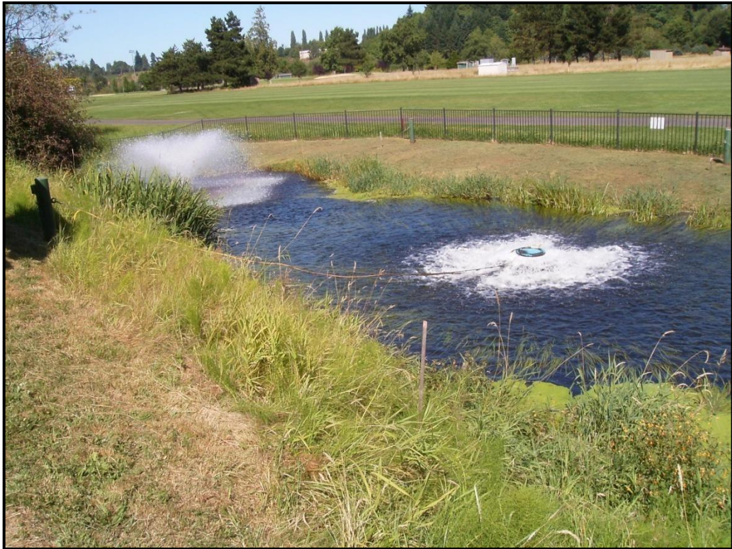
PHOTO 33: Drain Pipe Treatment Lagoon, looking northeast, with golf course in background.
