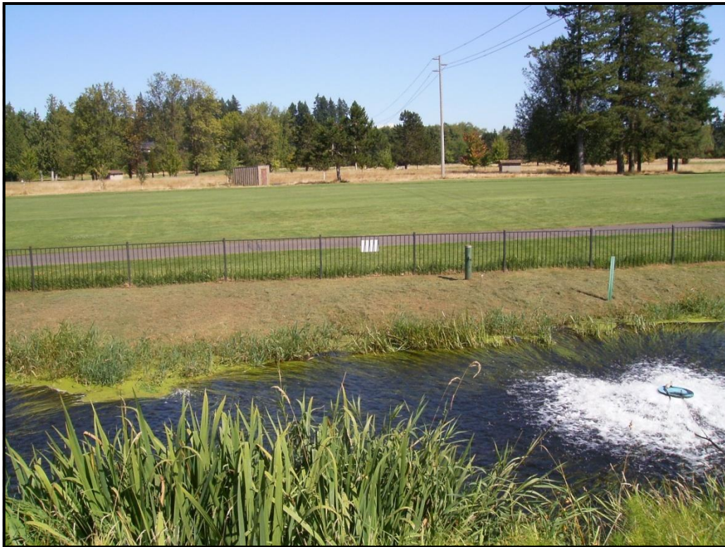
PHOTO 36: Looking east across Treatment Lagoon toward wells TW-20, TW-23 and TW-24.
