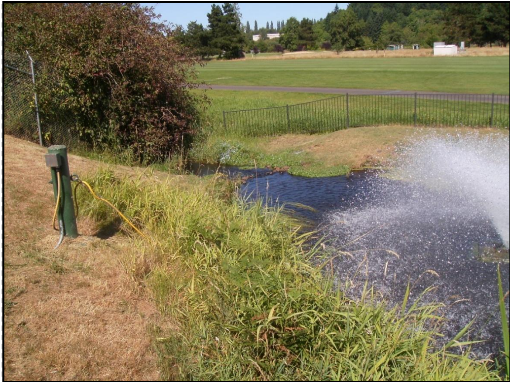
PHOTO 35: Looking northeast toward downstream end of Treatment Lagoon drainage feature.
