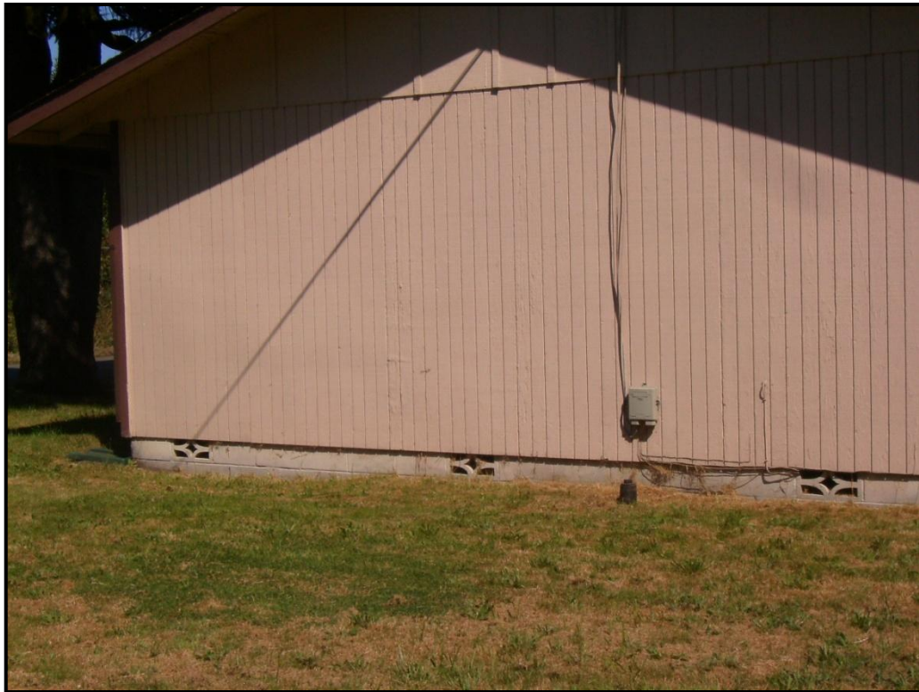
PHOTO 20: Typical residential perimeter foundation with crawl space; note crawl space ventilation.
