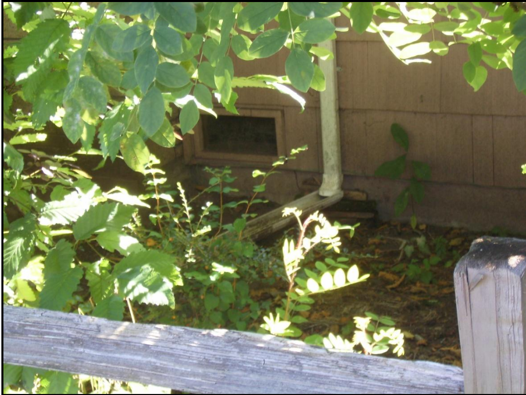
PHOTO 21: Close-up of residential foundation showing crawlspace ventilation.
