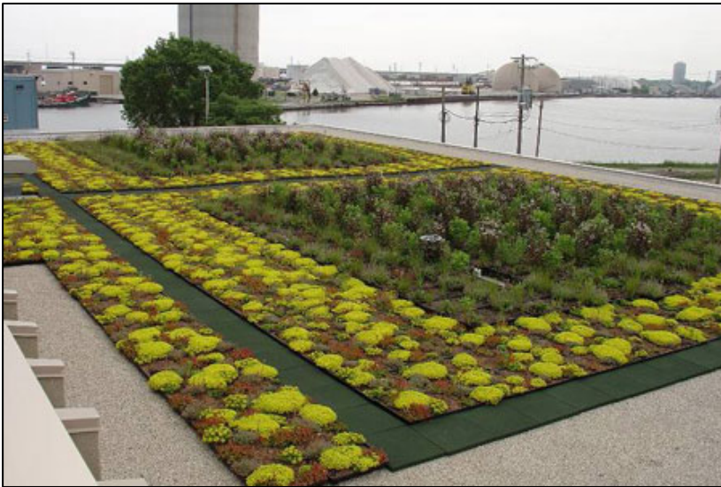
Green roofs such as this one in Wisconsin help filter rainwater, cool buildings and provide added green areas.
