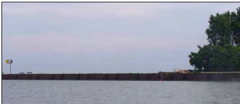
A bulkhead near the mouth of the river.
