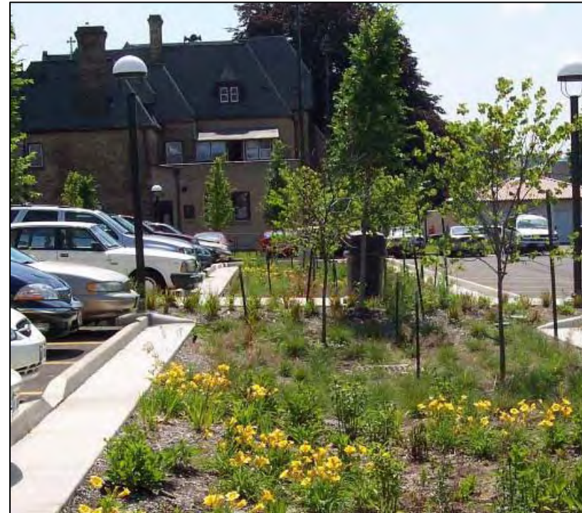
Bioswales are constructed areas filled with permeable soils and native plants, they help control and treat stormwater runoff.
