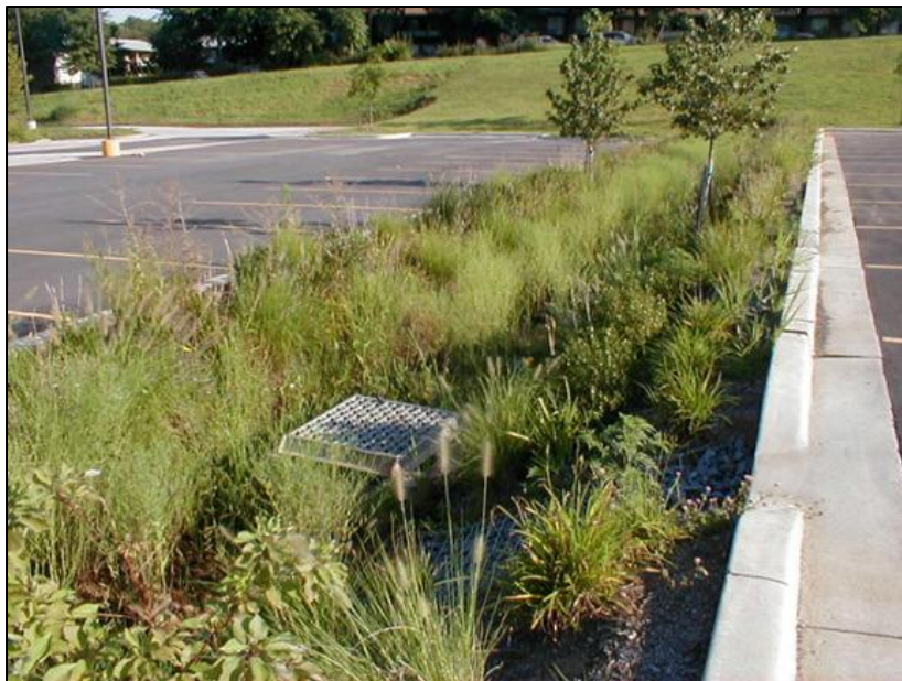
Well designed Bioswales provide a mechanism for infiltration and filtering stormwater.
