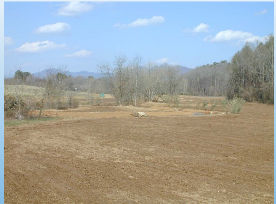
Stream restoration project immediately after construction; floodplain devoid of vegetation
