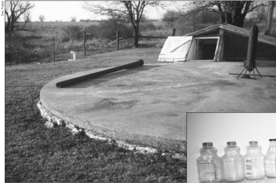
This dug well is vulnerable to contamination from nearby farming and grazing. After rainfall, water from the well is cloudy and often contains microbiological contaminants. Water from this well must be filtered and disinfected before it can be considered safe to drink. The bottles contain water taken from the well after rainfall.
