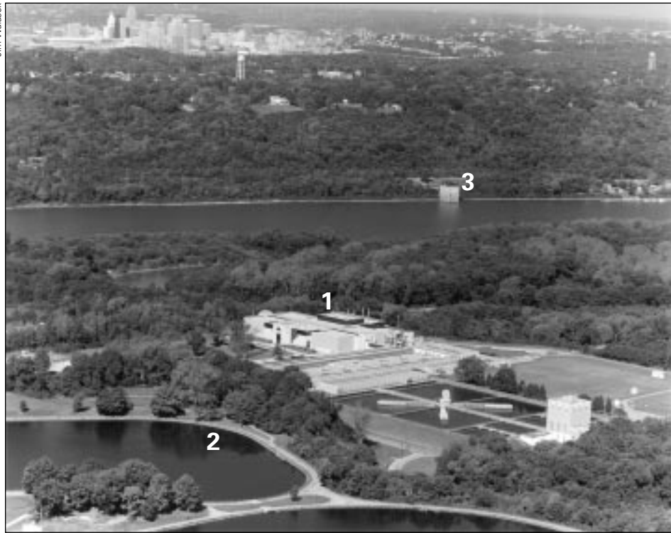
Cincinnati's surface water treatment plant was upgraded in 1995 to include deep bed carbon filtration. This process removes organic contaminants found in Cincinnati's source, the Ohio River. The treatment plant (1) and untreated water storage (2) are shown in the foreground. The intake (3) is shown on the opposite bank of the river. The city and elevated finished-water storage tanks can be seen in the background.
