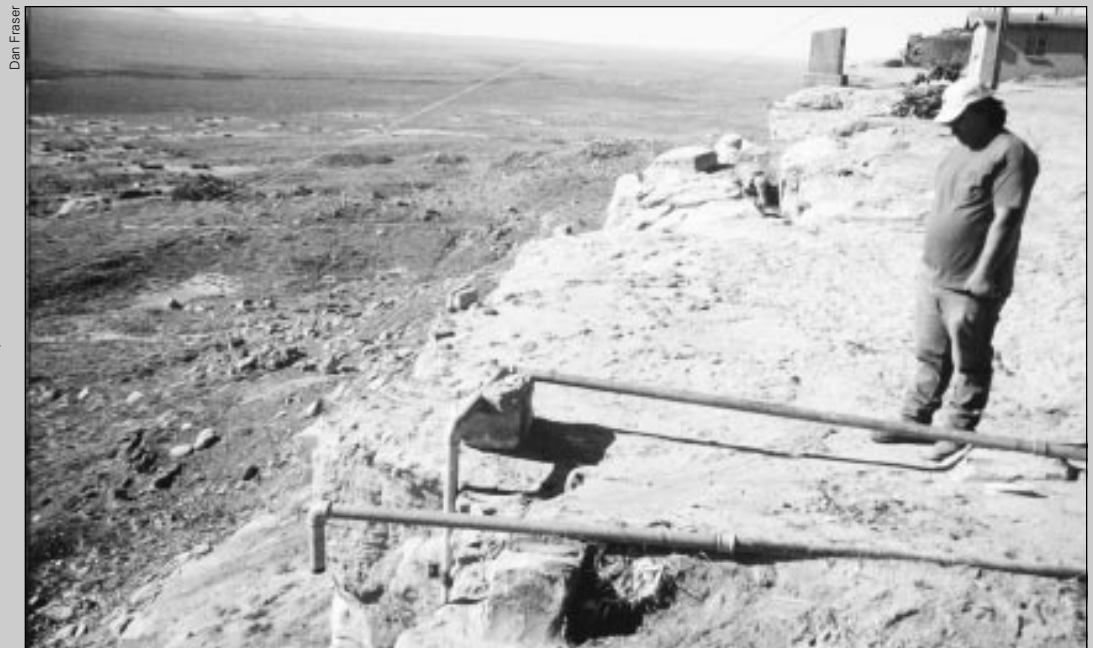
Chuck Villa, water system operator, looking down at the exposed transmission main ascending the face of the cliff.
