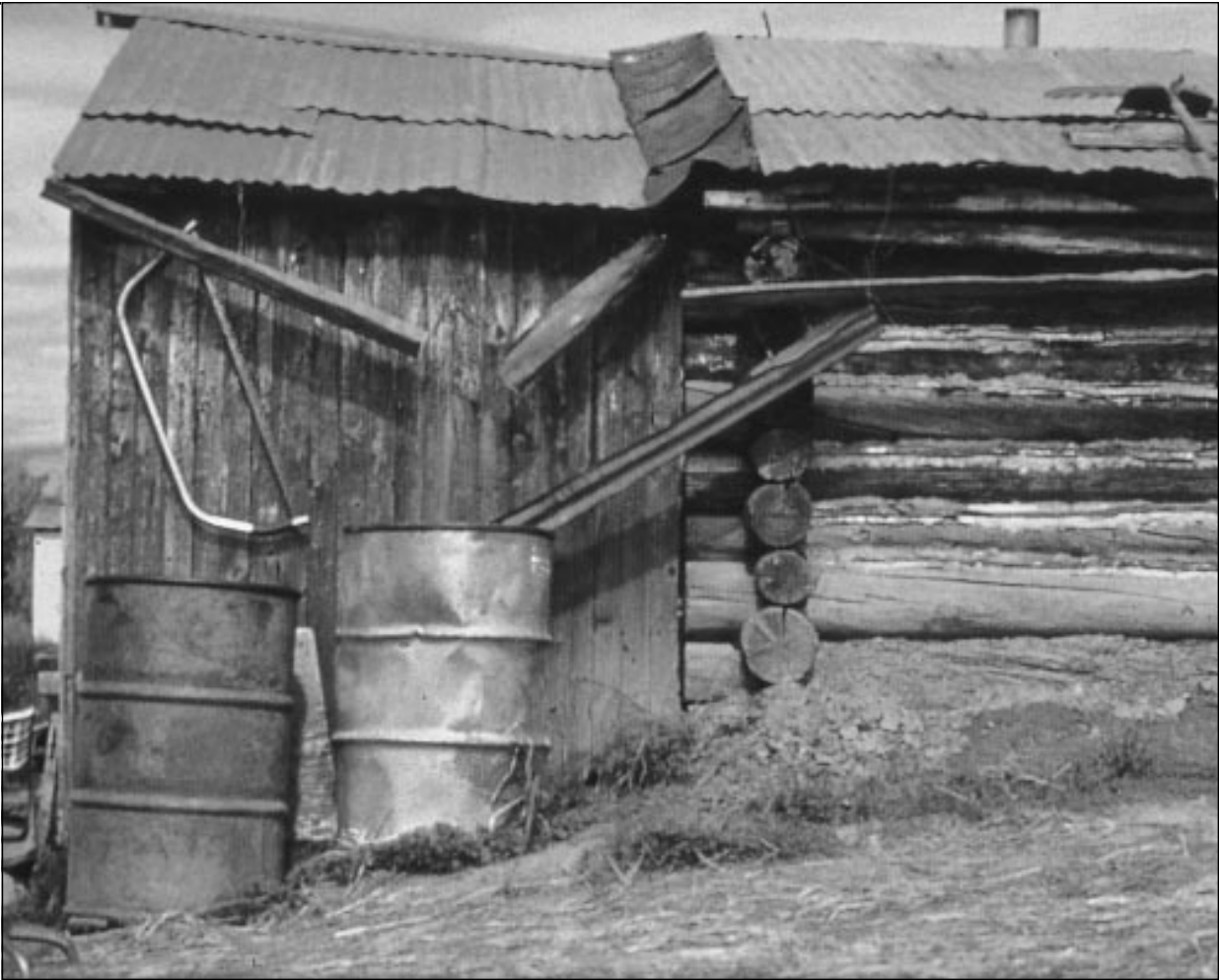
Rudimentary roof catchments provide drinking water for some households in the United States.
