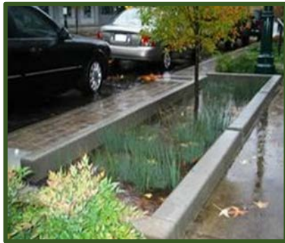
In-ground planter box, a type of green infrastructure technology, along an urban street.
