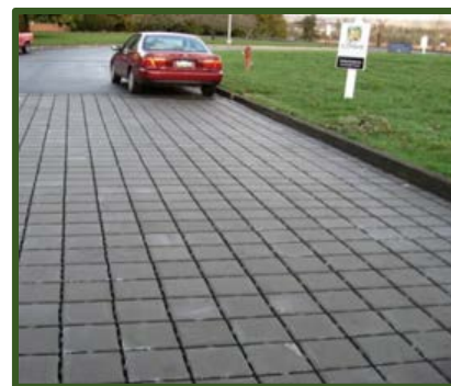
An urban street with permeable pavement, a type of green infrastructure technology.
