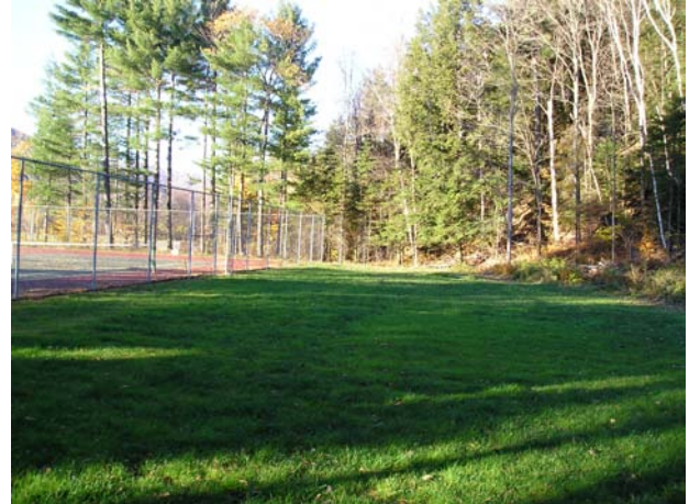
The dispersal field for the Warren Elementary School I/A system, three years after the system was installed.
