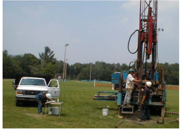
Installation of deep monitoring wells at Brooks Field.
