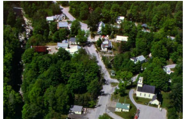
An aerial picture of Warren Village, looking north. The Mad River runs along the left-hand side of the photograph.
