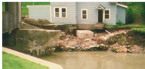
One example of an onsite system in the Village damaged by the 1998 flood event.
