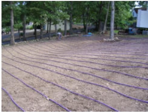
Drip tubing installed ready to be covered
