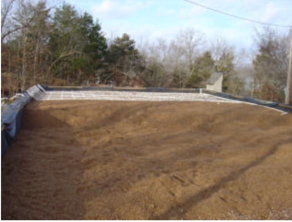
New gravel being installed during repair
