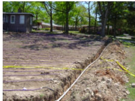
Drip tubing installed on top of existing soil.
