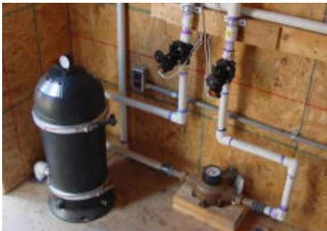
Effluent passes through sand filter
