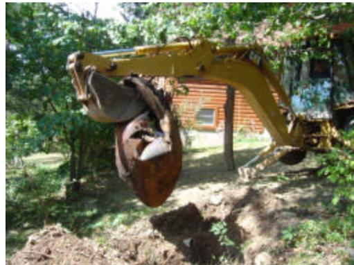
Rusted metal tank removed from ground
