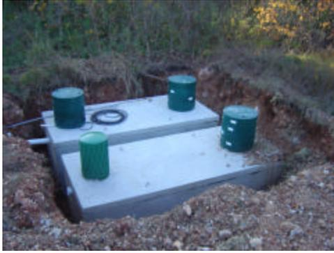
Treated effluent flows to 2 pump tanks
