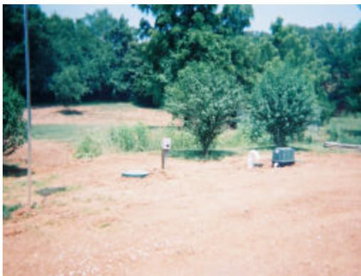
Air pump, tank vent, control panel and riser
