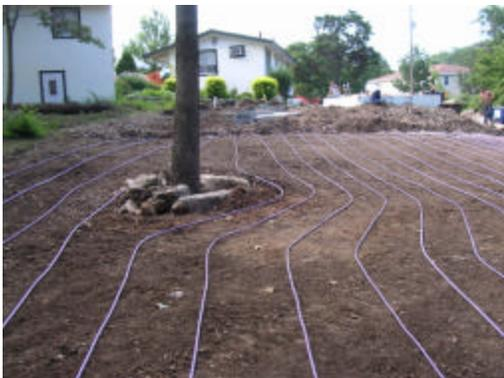
Flexible tubing allows for retention of trees
