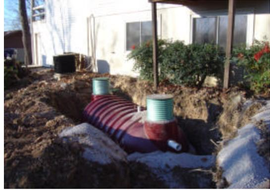
New fiberglass tank with advanced treatment installed
