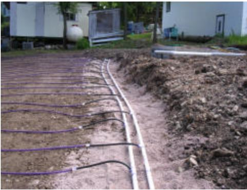
Tubing connected to supply and return lines
