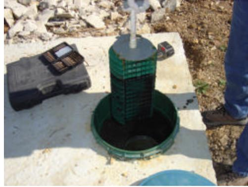
Effluent filter requires cleaning
