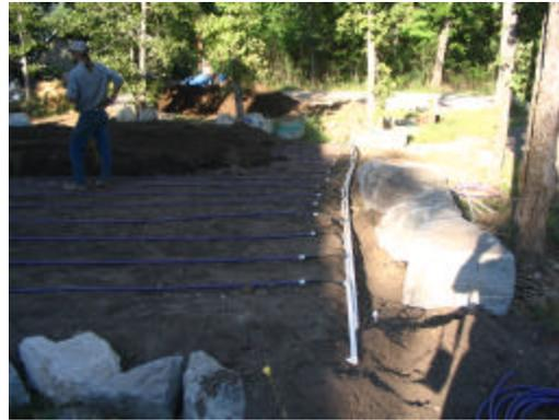
Treated effluent is pumped up to drip field
