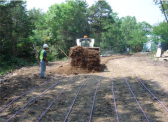
Drip dispersal lines installed on imported soil bed
