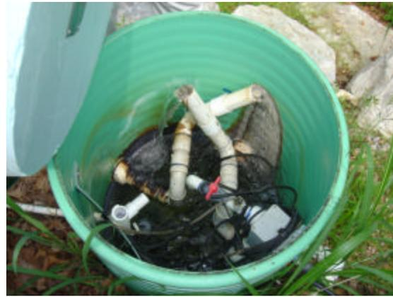
PVC pipes control water level in cells
