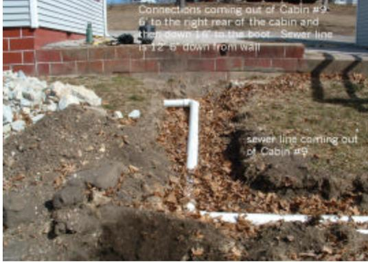
Sewage tank and filter tank installed and individual sewer line for resort cabin
