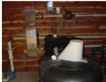
UV light disinfection and polishing by sand filter
