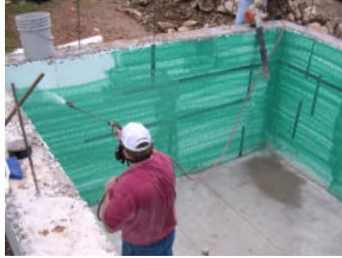
5,000 gal. drip dosing tank was poured in place.
