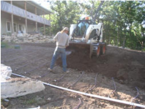
Imported soil placed over the drip tubing
