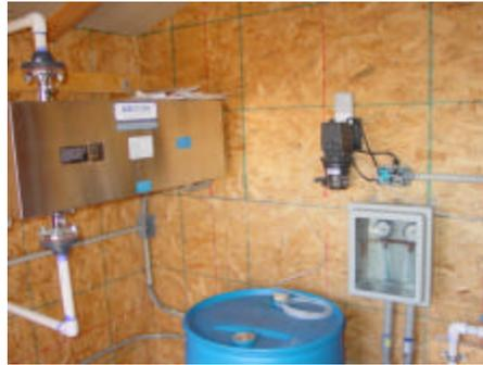
UV & chemical feed for phosphorus removal
