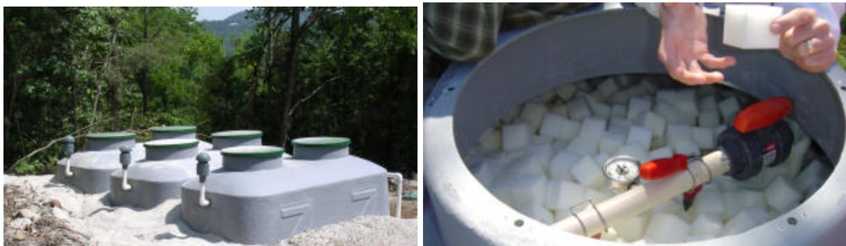
**Figure 3.5 ZABEL units and Foam cube filter.** Each lid opens up to a foam cube media filter and spray nozzle in the ZABEL wastewater treatment unit.
