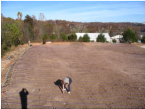
Drip tubing placed on bed of imported soil
