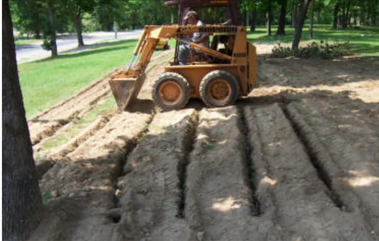
**Figure 3.7: Trenching in drip irrigation lines.** Adequate soil at this site allowed drip lines to be installed directly into the existing soil.
