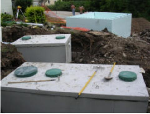
Concrete septic and treatment dosing tanks.
