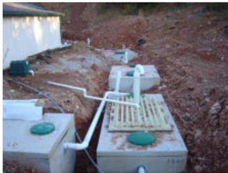
Grease trap, 2 septic tanks and treatment
