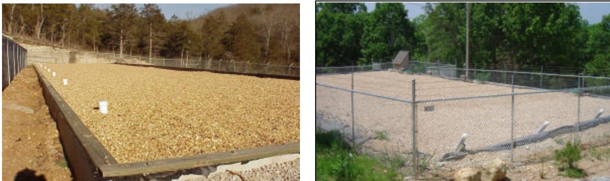
**Figure 3.6: Recirculating sand filters.** Large systems like the ones pictured can treat wastewater from a subdivision or housing complex.
