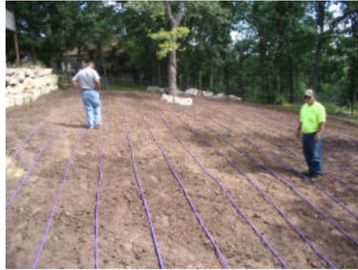
Drip tubing installed on imported soil
