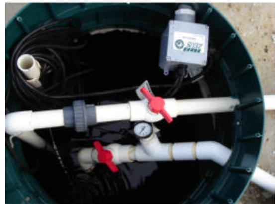
**Figure 4.2: Typical septic tank effluent and treated effluent sampling locations**
