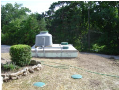
Treatment unit installed on the dosing tank
