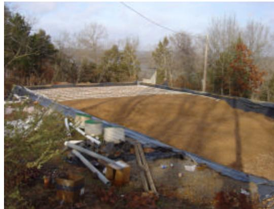
New gravel and piping with new liner in place
