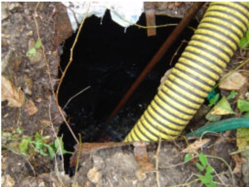
Pumping tank through rusted out lid
