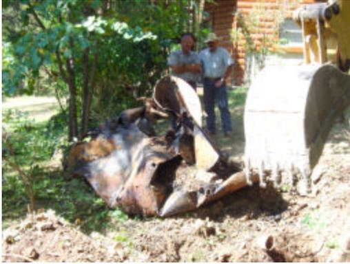
Effluent left tank through rusted out bottom
