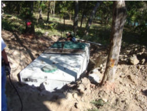
Tank hole enlarged with dynamite due to rock
