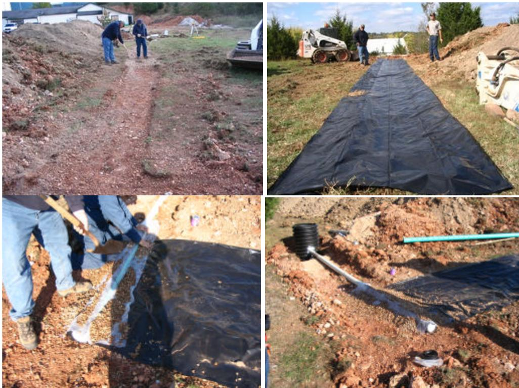
**Figure 4.5: Photographs of plastic sheet lysimeter installation**
