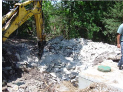
Setting tanks required rock removal
