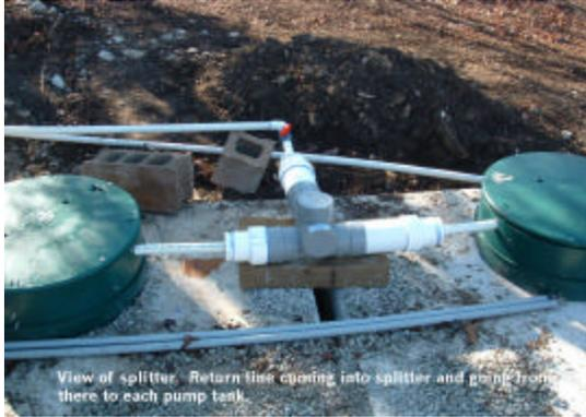
Septic and aeration tanks with dispersal and return lines for drip irrigation
