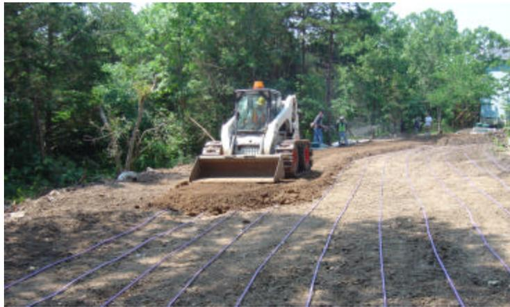
**Figure 3.8: Imported soil for drip irrigation lines.** Lines can be installed between soil bed and covering layer in imported soil.
