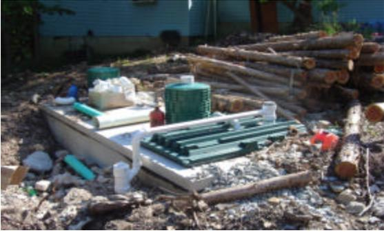
New concrete septic tank with treatment unit
