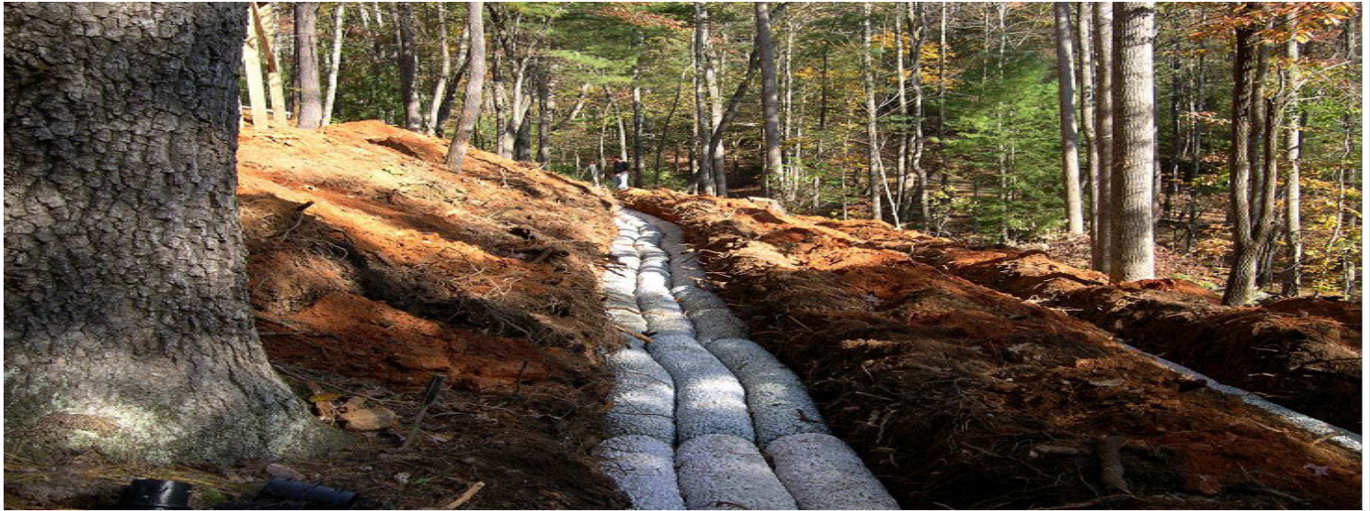
Installation of a non-gravel system in North Carolina
