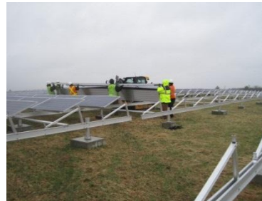
Installing solar panels
