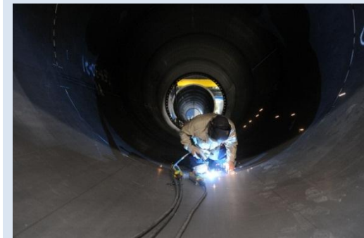
Venttower Industries employee welding on a wind turbine tower
