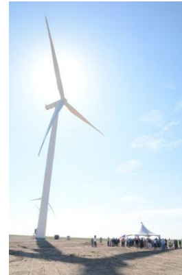
Officials celebrating PREP's ribbon-cutting are dwarfed by one of its turbines. Photo Credit: B&W Pantex
