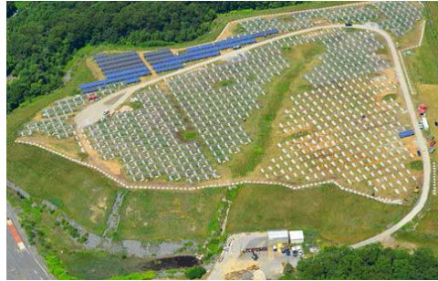
Scituate Landfill solar under construction, photo courtesy Brightfields Development LLC
