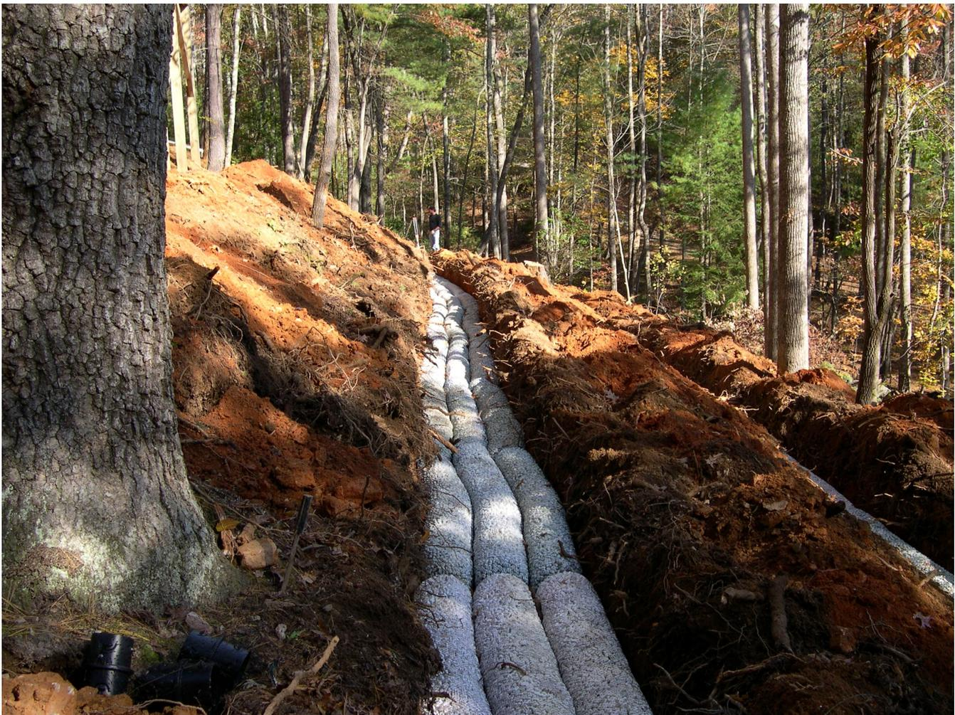
Non-gravel systems, like this one on a slope, account for half of the onsite systems installed in North Carolina.
