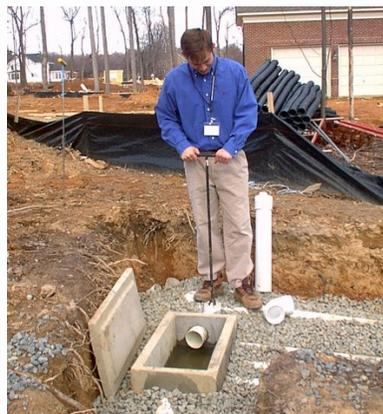
Fairfax, Virginia requires all new and repaired individual wastewater systems to install a flow diversion valve, like this one pictured, to allow the drainfield to dry out and avoid saturation problems.
