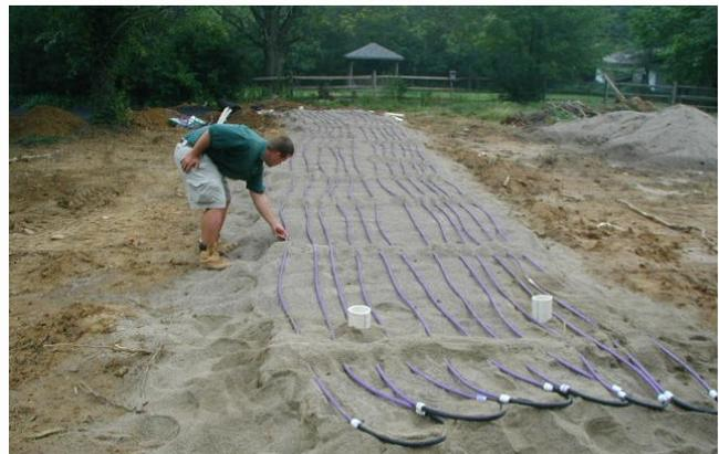
Sand filter systems, like this one being installed in Hamilton County, use sand to treat effluent. The effluent from the sand filter is then discharged, in pressurized doses, to a soil absorption bed.
