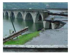
flooding and long-term river flow changes caused by climate change are expected to increase the frequency of bridge scour, further stressing the aging U.S. transportation system.
