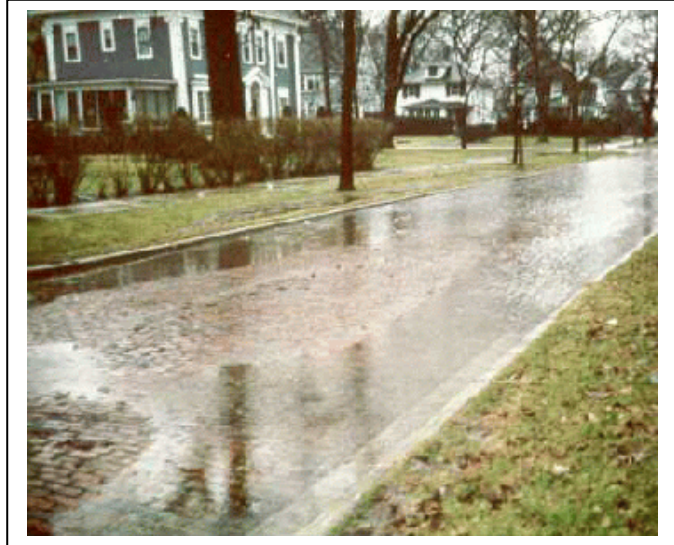
Figure 5.17: Runoff pooling on a street surface designed for temporary storage.
