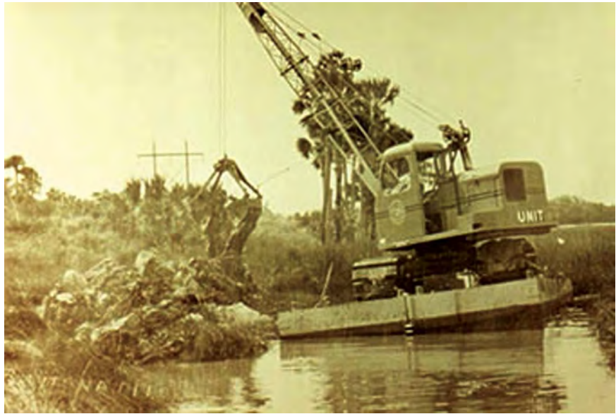
Figure 8. Historical mosquito control practice of using draglines to cut ditches through marsh areas. Source: Volusia County Mosquito Control.
