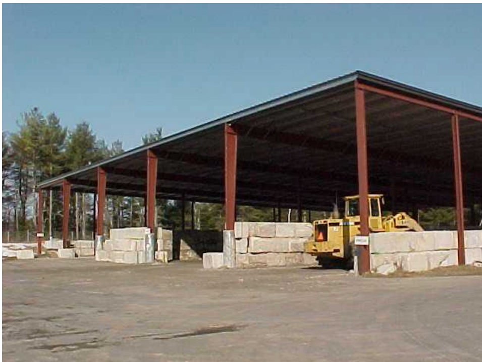
Figure 5-5. Permanent covered storage in Southern Maine (Courtesy Mark King, Maine Dept. Environmental Protection).
