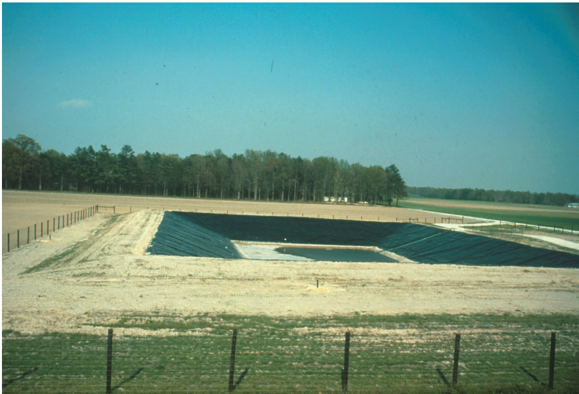
Fig. 5-5 A lined lagoon (Courtesy of BioGro Division).
