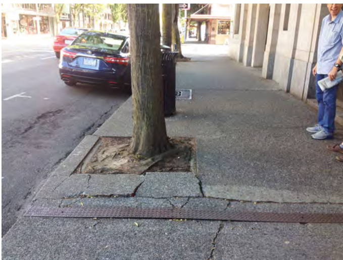
Figure 12: Many of the mature street trees downtown are buckling the sidewalk, causing unsafe conditions. (Image Credit: Urban Rain | Design)
