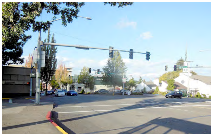
Figure 41: Existing view of the intersection of Capitol Way and 11th Avenue. The wide street, long waits for a walk signal, and numerous places where vehicles could potentially hit pedestrians make walking and bicycling unsafe. (Image Credit: Makers)
