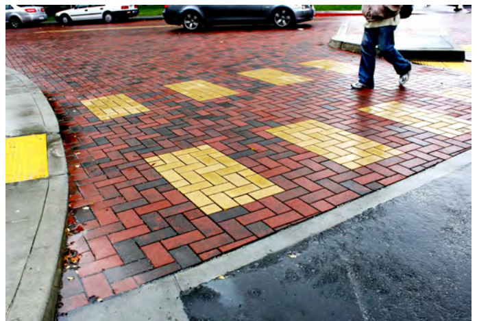
Figure A-6: Pervious pavers can collect and treat stormwater runoff. (Image Credit: Community Design + Architecture)
