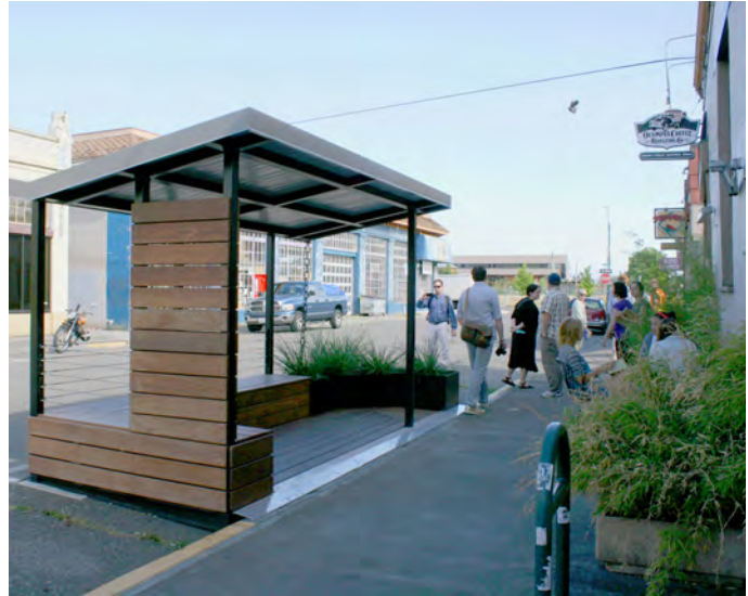
Figure 15: The parklet outside the Olympia Coffee Roasting Company in downtown Olympia provides a canopy to protect people from rain and sun and capture rainfall, which flows into the integrated planters. (Image Credit: Community Design + Architecture)
