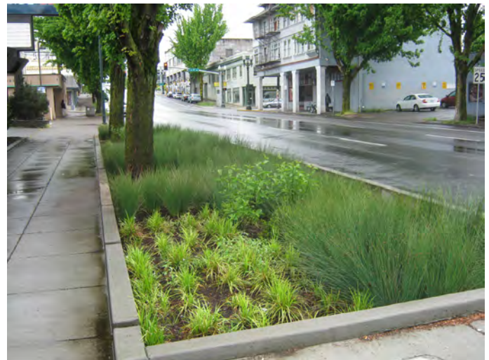
Figures A-3 and A-4: Before and after views of the Burnside/Couch curb extension stormwater planters in Portland, which show how stormwater management and treatment can be retrofitted into city streets with existing trees. (Image Credit: Urban Rain | Design)
