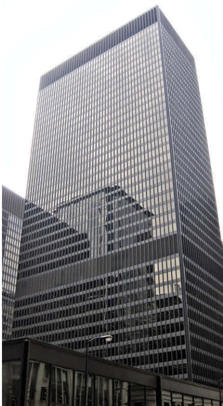
The Office of Personnel Management Nationwide Testing and Oversight Groups are located in the John C. Kluczynski Federal Building in Chicago.
