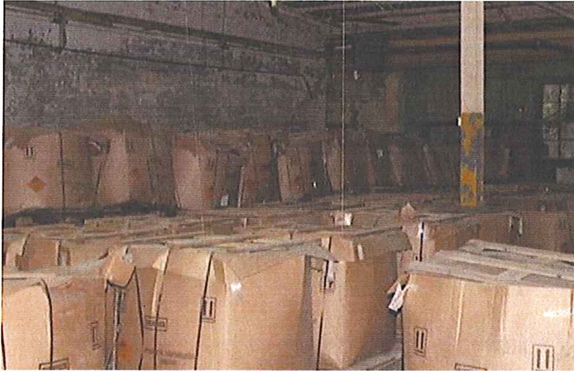
M6 Propellant in 880 lb bulk pack, Bldg 1610 (typical)
