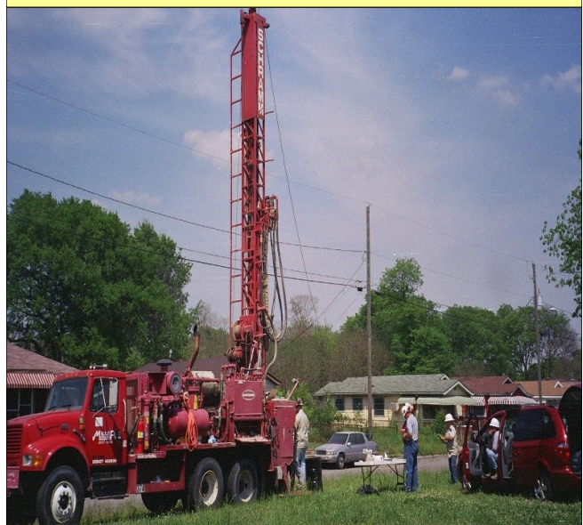
Example of drilling equipment installing a groundwater monitoring well.
