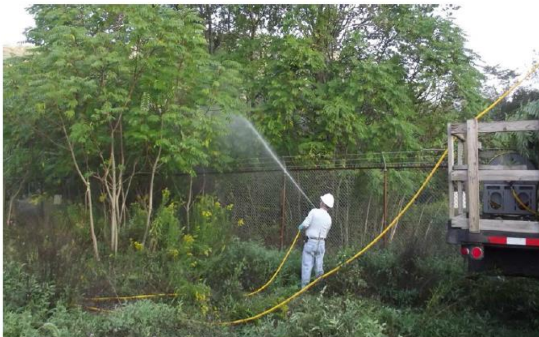
Figure 2: Dragging handgun and hose in Transmission/Distribution ROW
