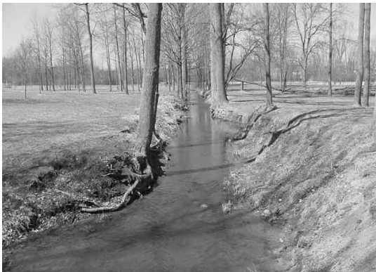
Firefighters Park Streambank Stabilization Before
