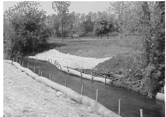
Firefighters Park Streambank Stabilization After
