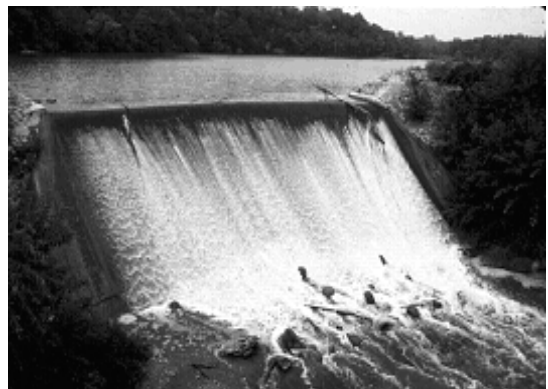
Phoenix Lake Dam
