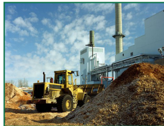
The McNeil Station biopower facility in Burlington, VT
