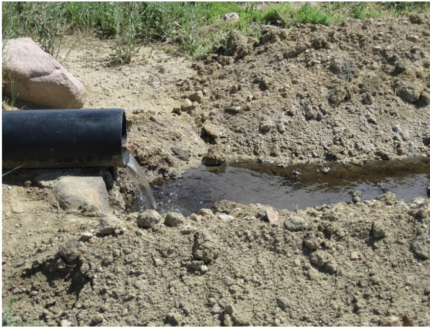
Figure 3 - Outfall 001 - SW Corner of Wastewater Holding Pit #2
