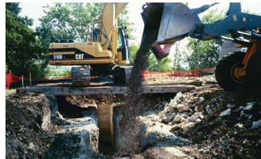
Media Backfilling of Biowall Trench
