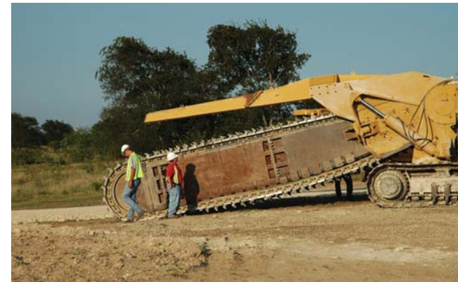
Trenching Machine Used in Biowall Construction
