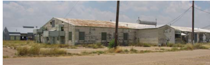
Formerly Used Military Building
