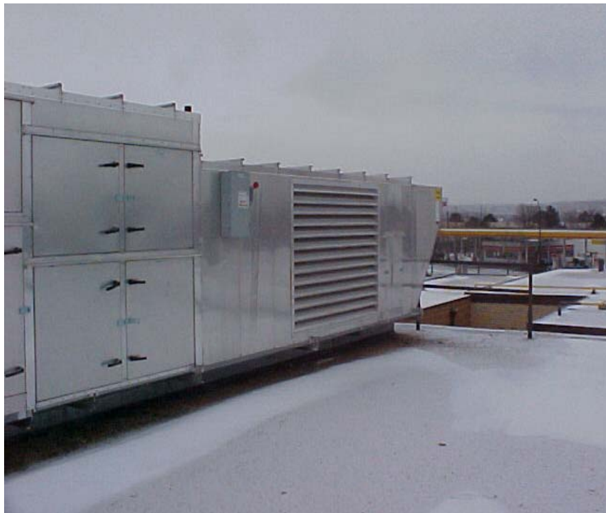
Roof Top HVAC Unit with Fresh Air Make-Up
