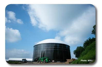
"This is one of the largest digesters on a college campus in the country. It'll generate 400 kilowatts of electricity every hour, which is enough electricity to power roughly 250 houses. To give a campus perspective, the digester could completely power Holmes Hall."
