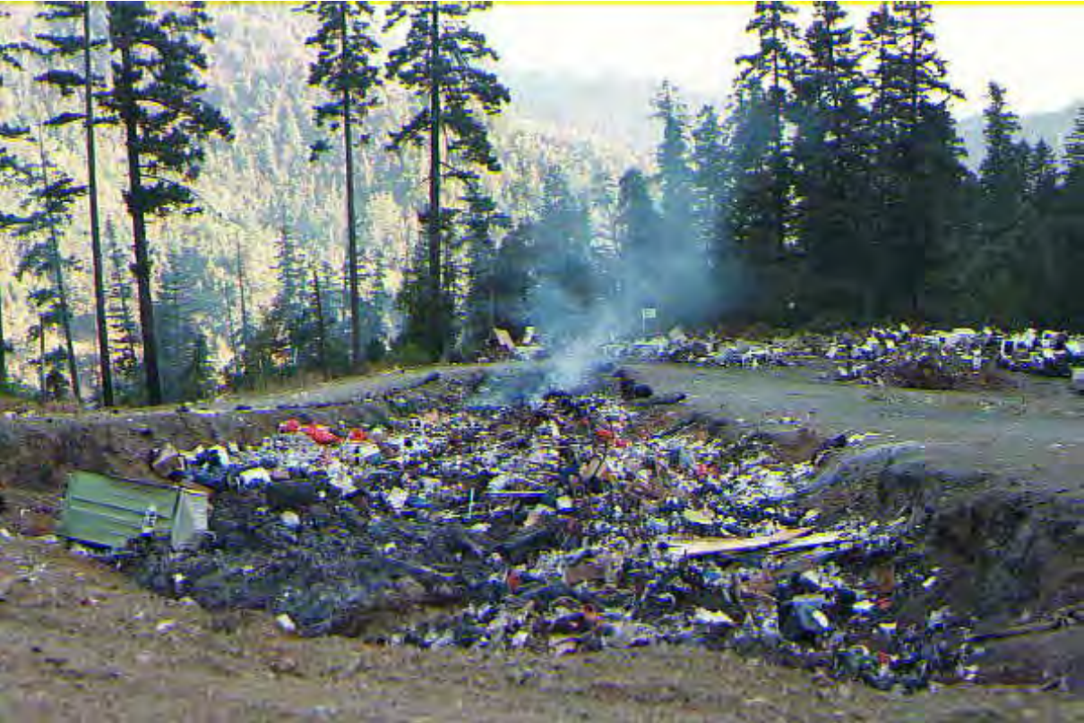
Supply Creek Landfill Prior to Closure (1997)
