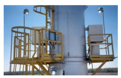
Figure 5. Continuous Emissions Monitor. These instruments provide high quality information on air emissions and exhaust gas characteristics. See Recommendation 1.1.
