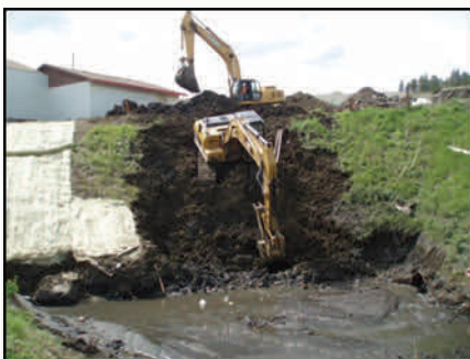
Excavation above Sundance Creek
