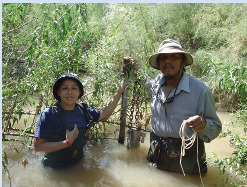
Gila River Indian Community YSI Sonde installation for continuous water quality monitoring at the Pee Posh Wetlands. Photo courtesy of Gila River Indian Community.
