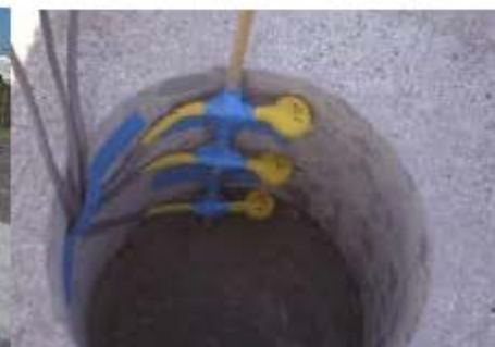
Embedded Thermocouples
