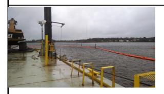
Portion of silt curtain dislodged from the pylon
