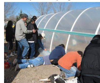
Raising a hoop house for a school class gardening project.
