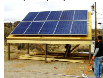
A homeowner found help within the community for a solar-panel installation.
