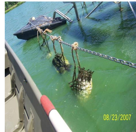
Stormwater Pond With SolarBee & Floc Logs
