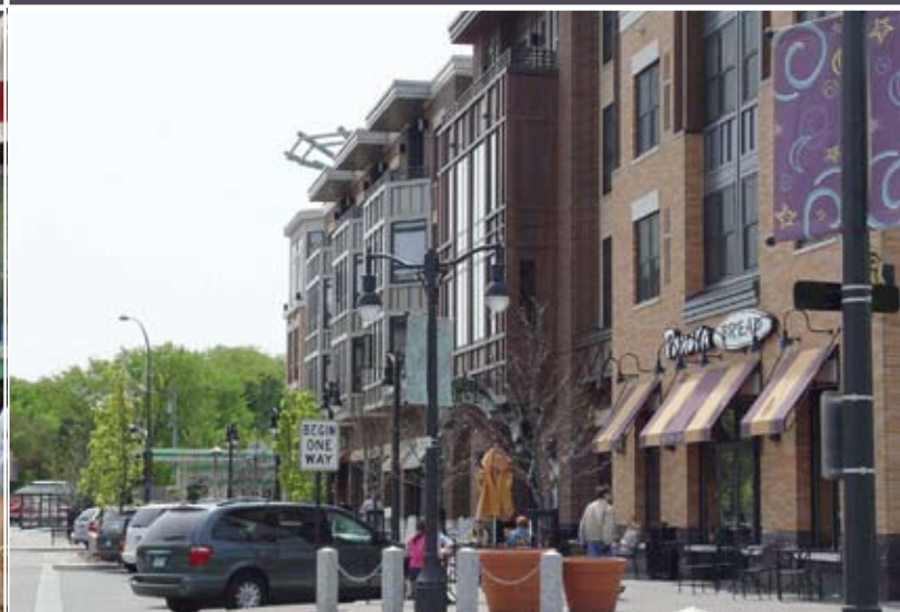
Strategic public investment helped to create this walkable town center for St. Louis Park, adding stores, housing, services, and a new town green.
